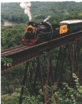
The steam engine at the Boone & Scenic Valley Railroad pulling passengers across the mile high bridge.
